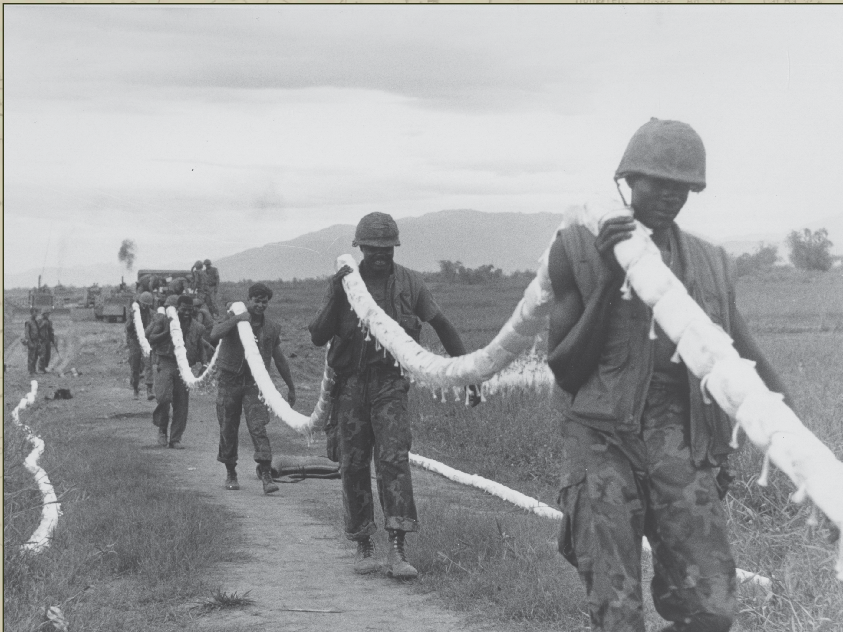
A U.S. Navy Mobile Construction Battalion (Seabees) lays explosive lines to clear a route of buried mines to construct roads in South Vietnam, September 1970. By 1972, as news of the riots aboard the Kitty Hawk and Constellation spread throughout the Navy, it awoke underlying racial tensions between Seabees at Naval Station Midway Island leading to violence between black and white Seabees. (Navy History and Heritage)
